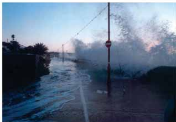
Figure 2. Inland flooding – overtopping and flooding at St Aubin's sea wall near the Gunsite slipway
