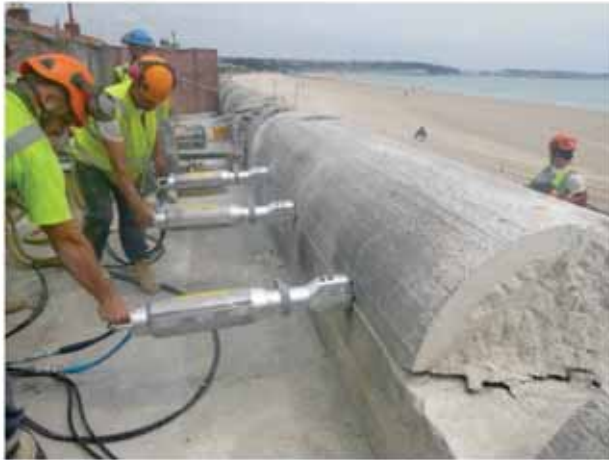
Figure 11. Concrete splitters removing the top of rounded wall
