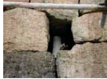
Figure 17 - Anchor expanded
