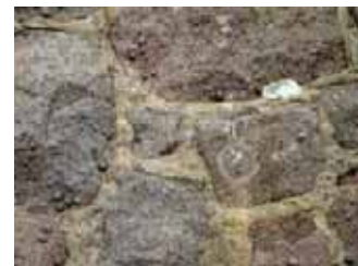
Figure 20 - Anchor with plug cap replaced, 'Secret Fix'
