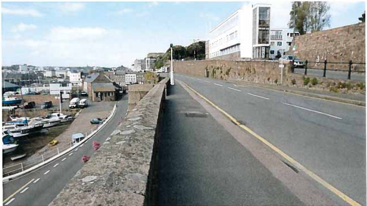
Fig 4. View looking up
