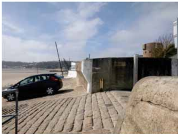
Figure 9. Gunsite angular recurve at the slipway
