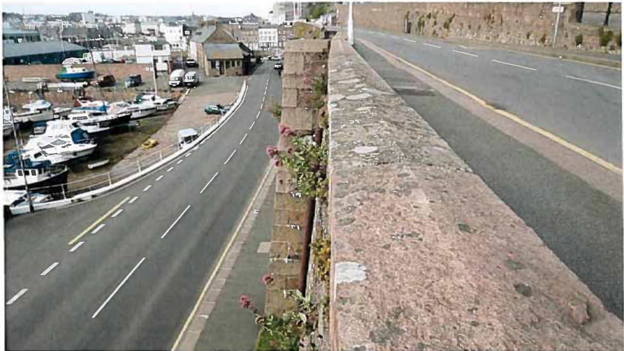
Fig 5 View looking up
