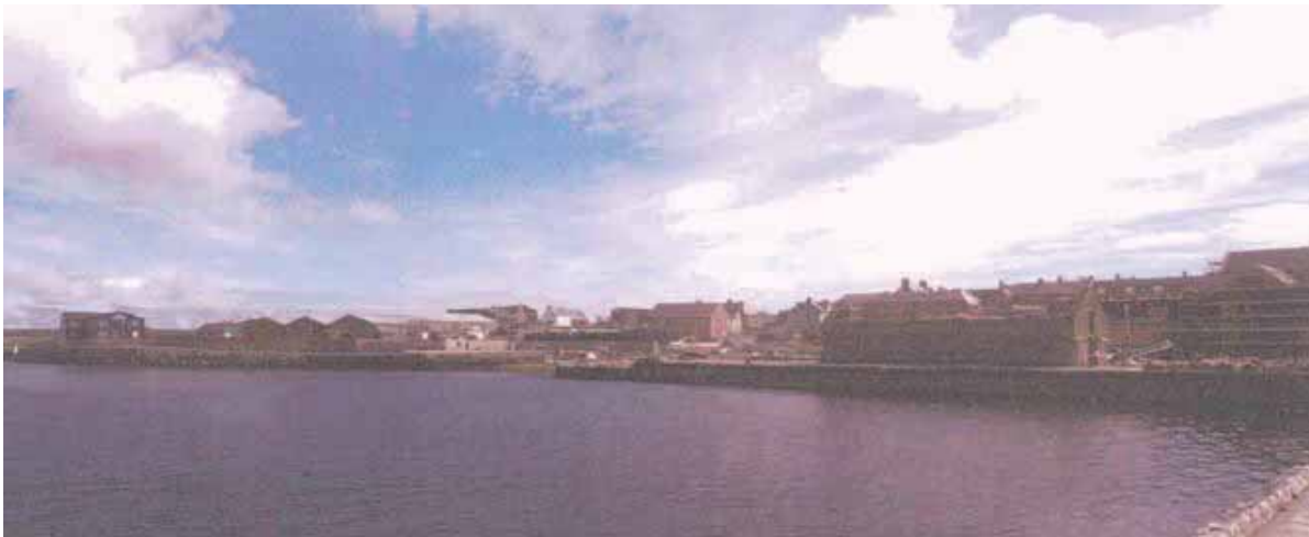
Panorama of Hay's Dock with the Heritage Centre under construction in the background (right), the restoration of the old sail house on the quay (centre right) and Cintec stabilisation work (end of the quay left of sail house).
