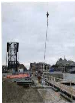
Cintec anchors hoisted into place by crane
