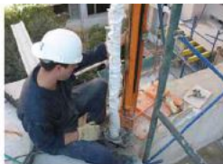
Anchor positions were carefully marked out and drilled with extreme precision to avoid intersecting anchors
