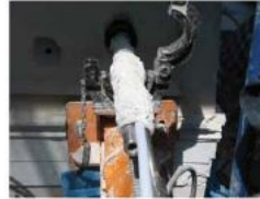
Anchor positions were carefully marked out and drilled with extreme precision to avoid intersecting anchors
