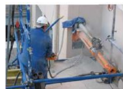
Anchor positions were carefully marked out and drilled with extreme precision to avoid intersecting anchors
