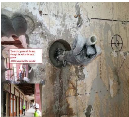
TYPE 1: Cintec No 8 Rebar 2205 (1" Dia) Reinforcement
