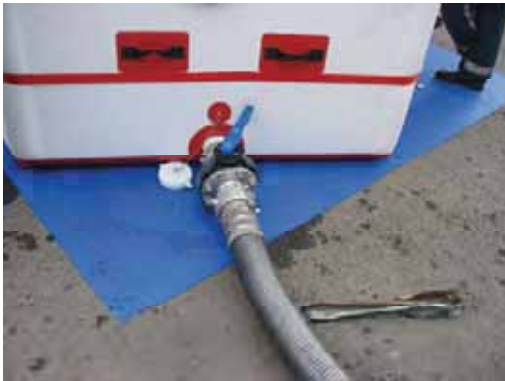
Attach suction hoses as required
