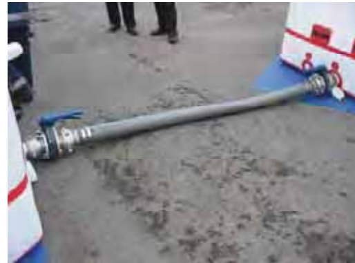
If two dams are to be deployed, join the two units with a short male-male suction hose
