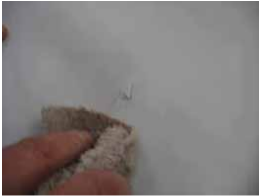
Thoroughly clean area around tear.
