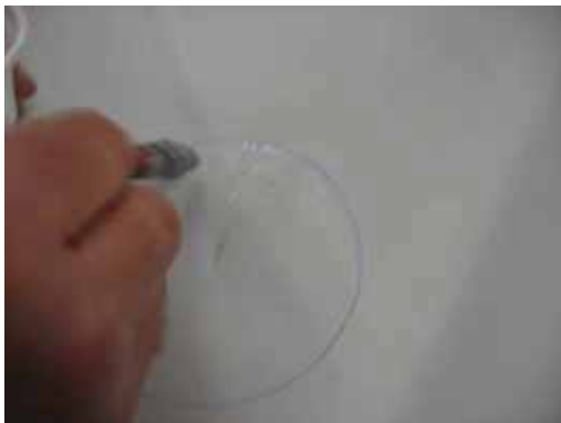
Apply glue within the marked area. Wait 20 minutes and apply second coat
