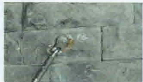
Upper Fixing Detail - Cintec Stud Anchor with Eye Nut attachment.
