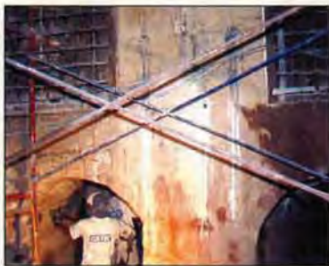
Drilling the vaults
