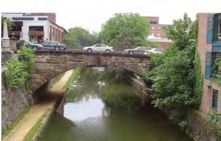
The Chesapeake & Ohio Canal flows under the stone masonry arch of the Wisconsin Avenue Bridge in the busy Georgetown area of Washington, DC. The towpath beside the canal serves as a footpath and recreation resource. The original wrought-iron railing dates back to 1831.
