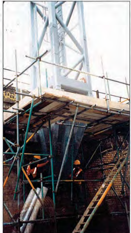
The torquing of the anchors
