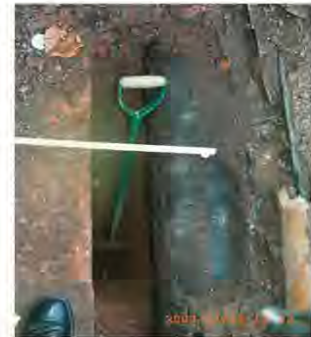
Fig 1. Excavations revealed a large gas main close to the north wall.
