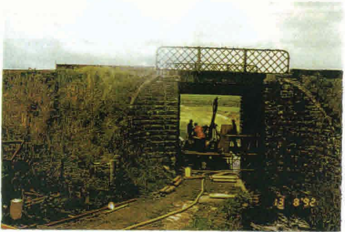
Installation of Ground Anchors Through Railway Bridge Abutment
