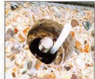
Anchor prior to injection
