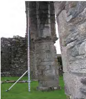
Image revealing the extent of wall and column rotation prior to stabilisation
