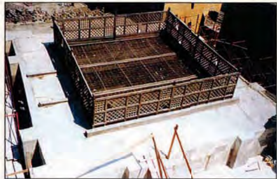
Roof section above central courtyard
