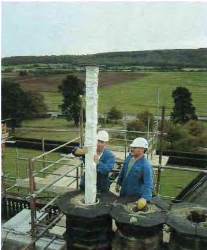
Chimney's capped with a stainless plate. ->
