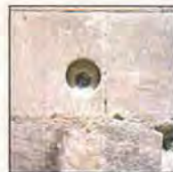
Anchor installed & inflated ready for front core to be replaced
