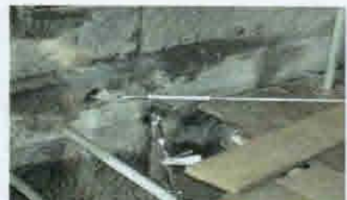
Lower fixing detail with turn buckles.
