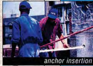
typical consolidation anchor prior to grout injection
