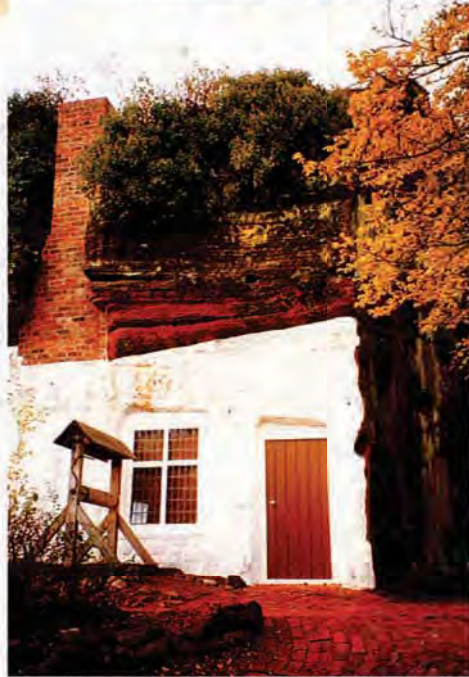
External view of main entrance to restored dwelling.
