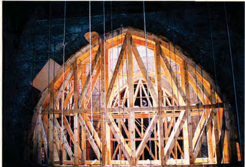
Temporary support of the Dikka arches
