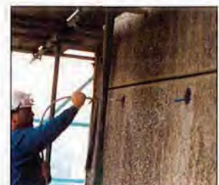
Injecting grout into anchor
