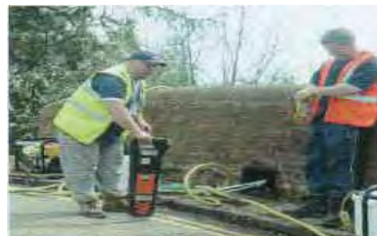
Checking for sub-surface services during bridge survey
