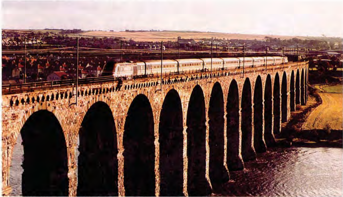
Royal Border Bridge, carrying London -Edinburgh mainline train. Photo : Mel Holley ©
