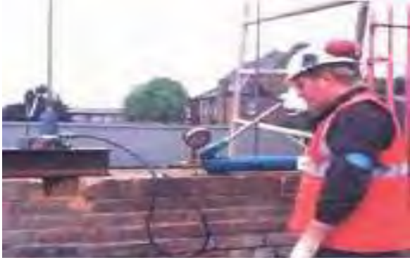
Post-Tensioning Cintec anchor in test panel..
