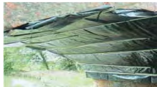
Temporary below arch protection during the installation process
