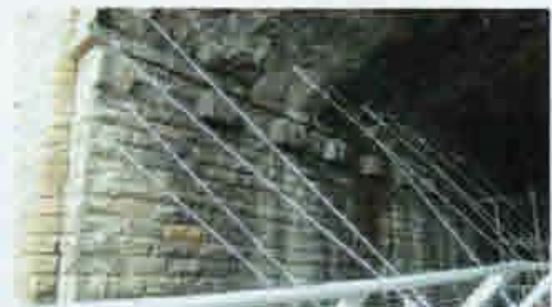
View of the supporting cables under the arch after lifting bridge from supporting scaffold.
