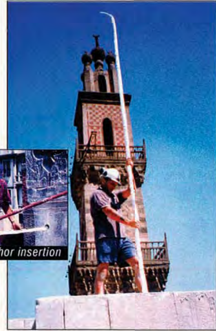
5 metre long vertical anchors at roof level
