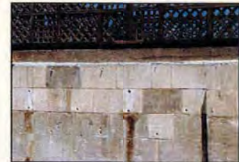
Roof consolidation anchors
