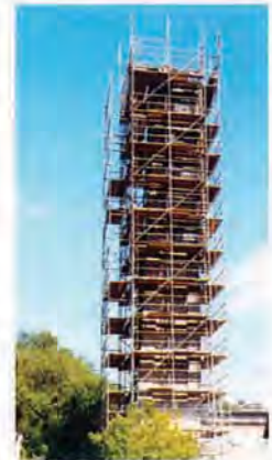
Chimney Restoration In Progress
