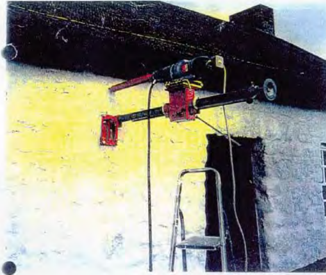
(b) Drilling Rig in place.
