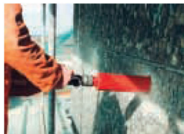
Diamond core drilling
