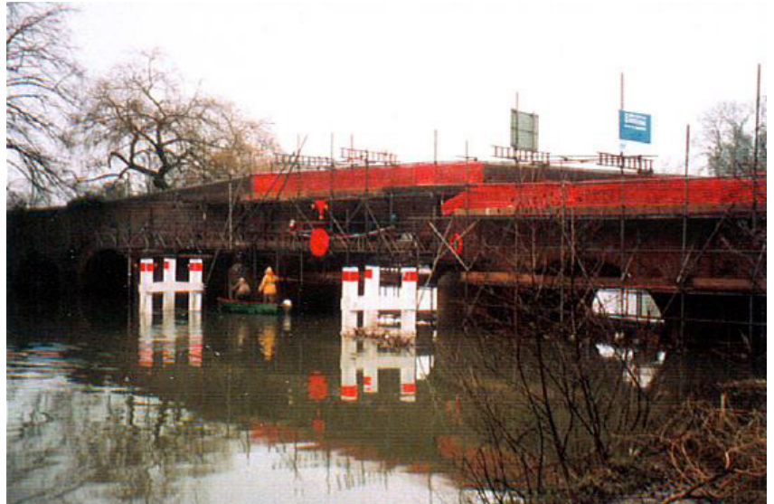
Historic Sonning Bridge at Reading
