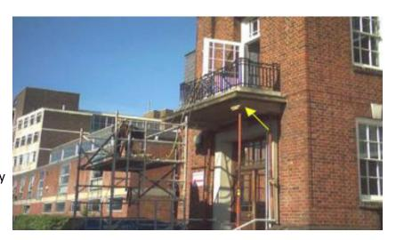
Technical Services Team devised a solution using Cintec anchors secured in TST Systems' profiled holes. It was calculated that this combination system would achieve the "pull- out" loads required to safely secure the balcony whilst overcoming the problem of inadequate material surface area to anchor to.
