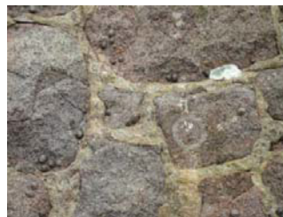
Figure 20 - Anchor with plug cap replaced, 'Secret fix'
