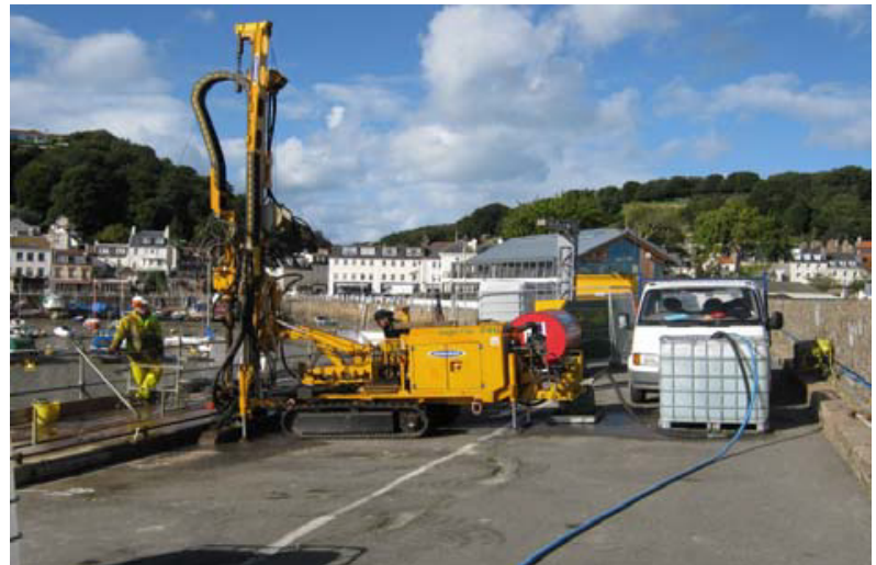
Figure 19 - North Pier vertical drilling
