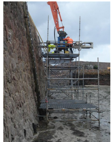
Figure 19 - Fort horizontal drilling
