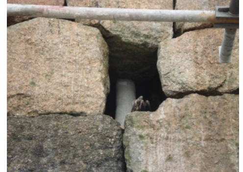
Figure 17 - Anchor expanded
