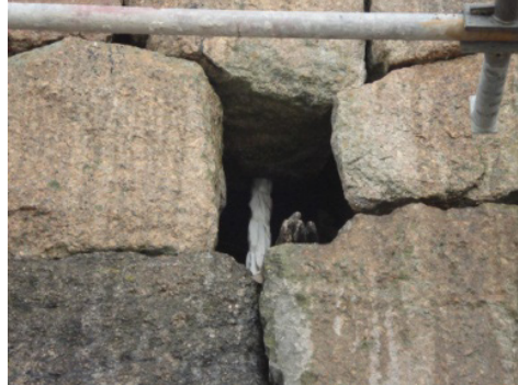
Figure 16 - Pre-injection with masking tape
