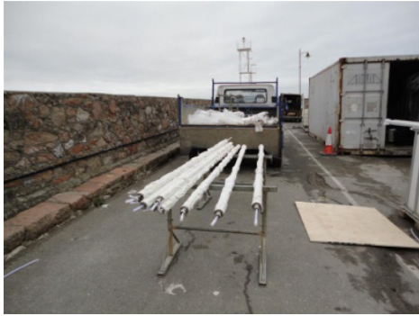
Figure 15 - Anchors with coupler
