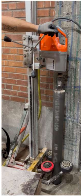
Core Hole Drilling
