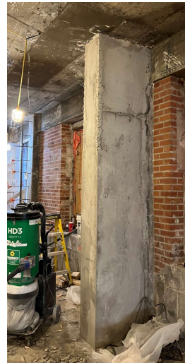
Structural dowels and rebar were installed within the formed and poured column
