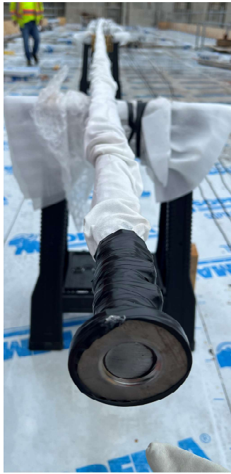
On-site Anchor Assembling
