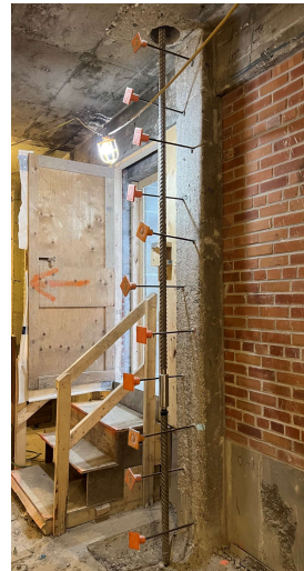
Structural dowels and rebar were installed within the formed and poured column
