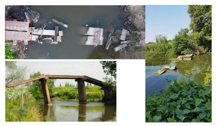
When Cintec visited the site in 2018 all that was visible of the remains of the bridge were random sections of stone beams partially or totally submerged in the river.
