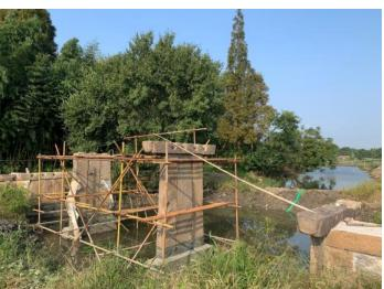
New foundations were formed in the river bed and pockets left to receive the repaired vertical members forming the piers. The horizontal and inclined stone members were then carefully placed and pieced together without the need for any mechanical connection as individual stones had original socket and tenon joints.
