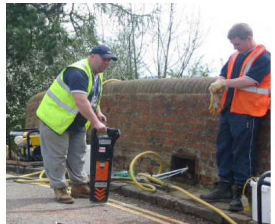
Checking for sub-surface services during bridge survey.
