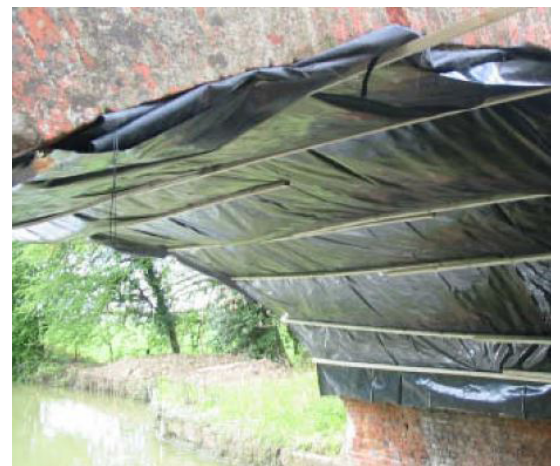
Temporary below arch protection during the installation process.
