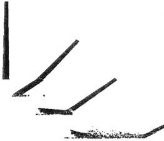
Figure 2.(a). Controlled demolition of a chimney.
