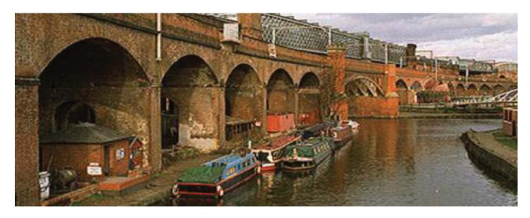
The busy Deansgate rail viaduct is situated in the heart of Manchester spanning numerous buildings, roads and canals. In 1997 the normal daily flow of rail-traffic was disrupted by a destructive fire which took hold in a workshop located directly underneath. The subsequent heat generated by the blaze caused extensive damage and a weakening of the seven rings of
