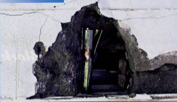
Figure 2 Substrate Drilling Damage
