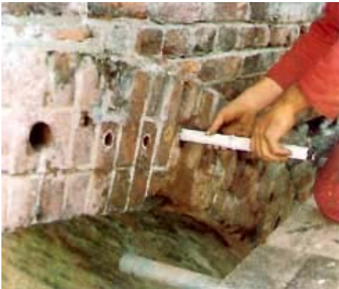
Placing the anchor in the prepared hole
