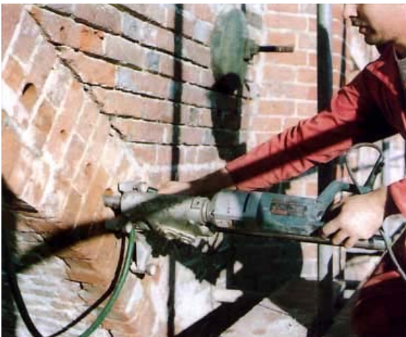
Core drilling holes for the anchors
