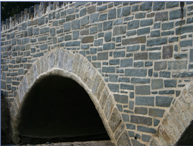
Century Lane Bridge, Buck's County, PA
