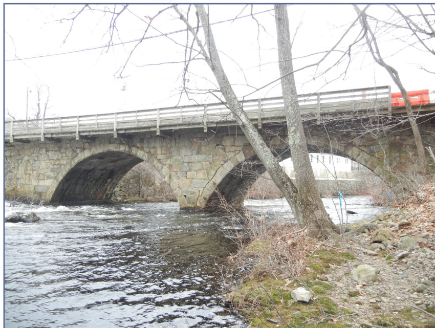
Slattersville Bridge, North Smithfield, RI
