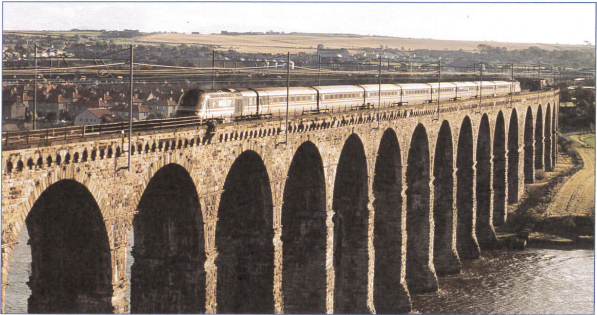
Royal Border Bridge, carrying London - Edinburgh mainline train. Photo : Mel Holley®
