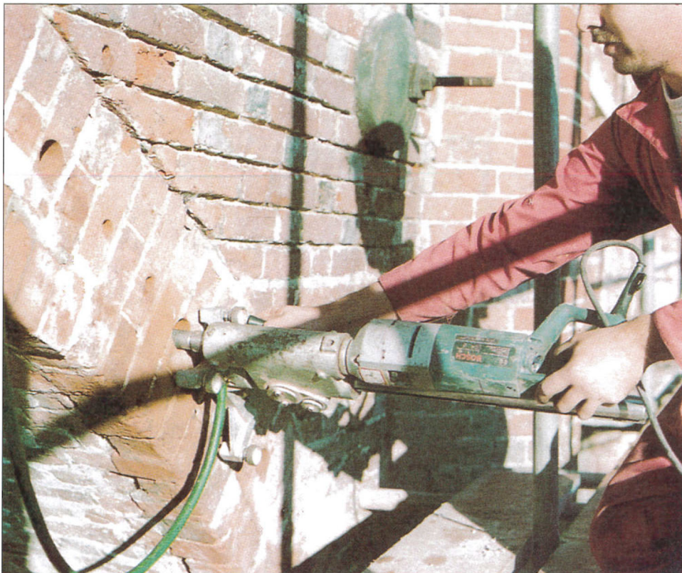
Core drilling holes for the anchors
