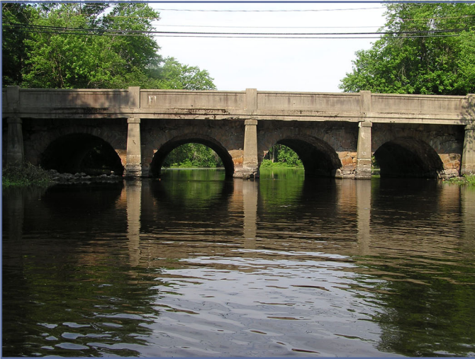
Ames St. Bridge, Dedham, MA
