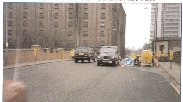
DUCIE BRIDGE - MANCHESTER
