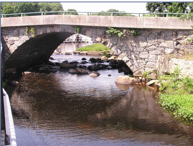
Harrisville Bridge, Harrisville, NH
