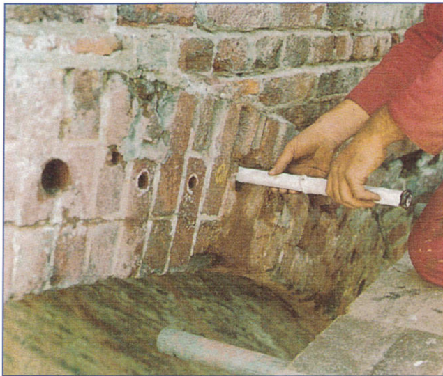
Placing the anchor in the prepared hole
