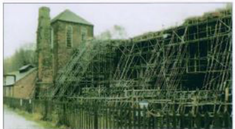
Restoration work in progress
