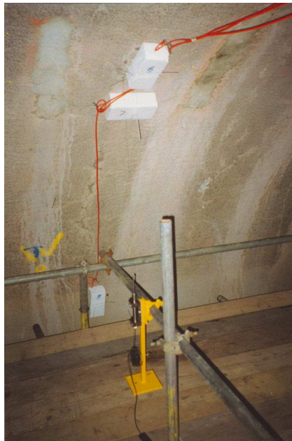
Figure 15 Deflection and Strain Instrumentation in Location
