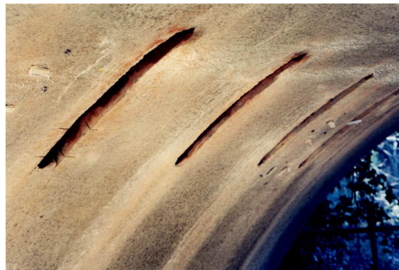
Figure 10 Installation of J-Bars
