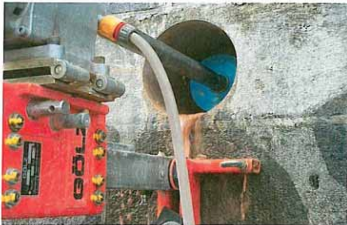
Core Drilling
