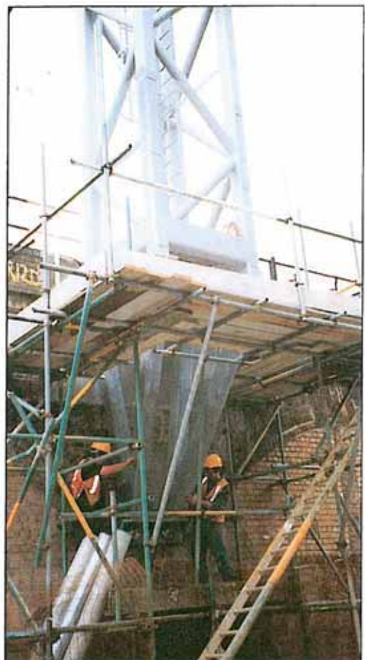
The torquing of the anchors
