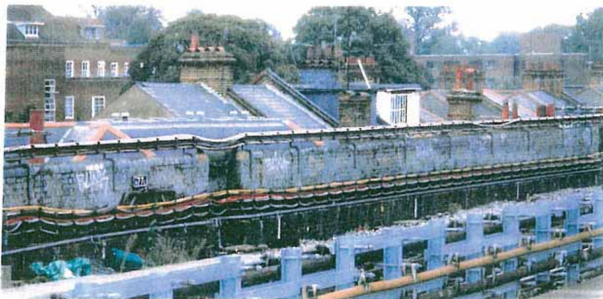
Figure 1 Parapet wall with bolted on utilities
