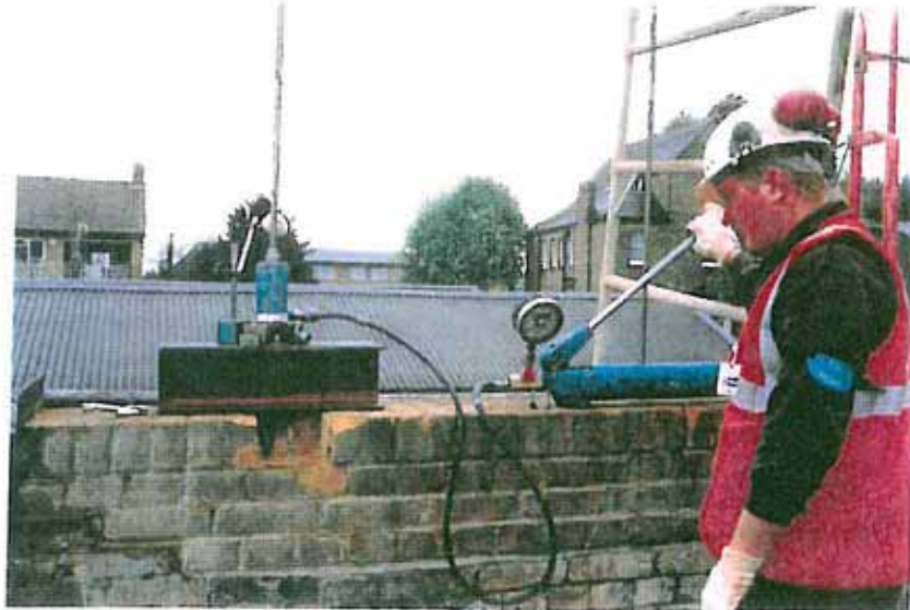
Figure 4 Post-tensioning Anchor in Test Panel
