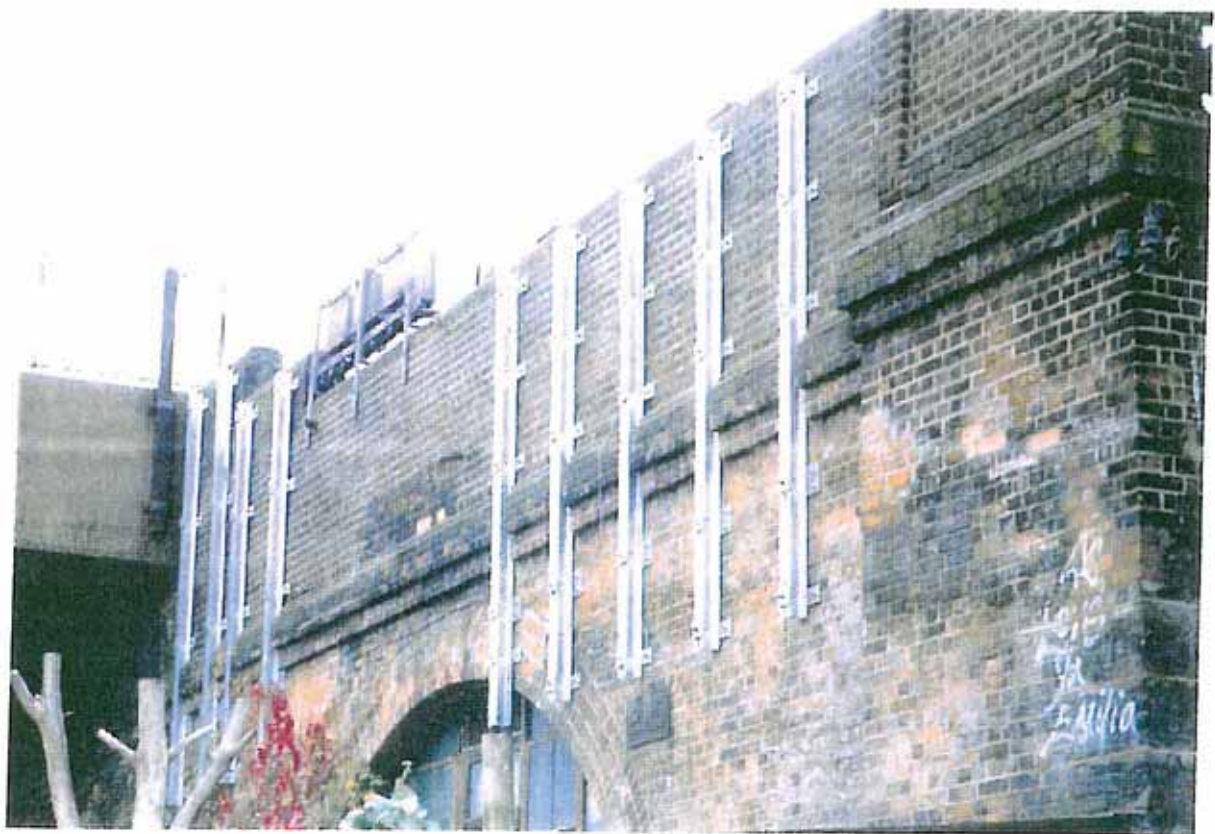
Figure 2 Externally strengthened wall
