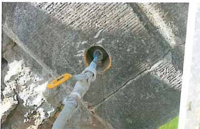
Anchor grout injection
