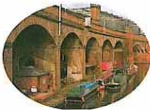
Bridge and Viaduct Reinforcement
